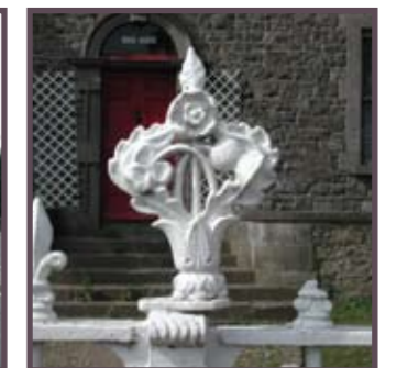
Fig.7: Detail from gates on the Octagon (courtesy of the National Inventory of Architectural Heritage)
