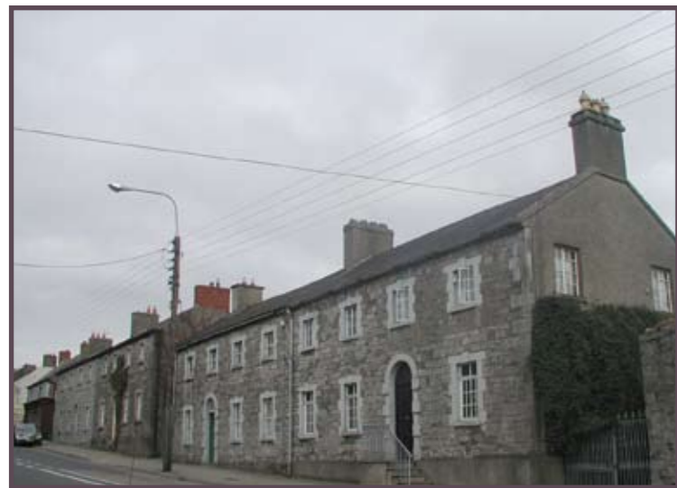
Fig.12: Range of stone facades to terraces on the east side of Chapel Street
