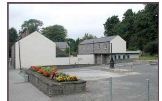
Fig.22: Car park & public toilets in an open space on Church Street.
