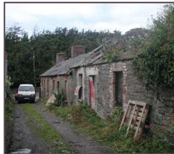
Fig.13: Range of derelict nineteenth-century estate cottages perpendicular to Chapel Street.
