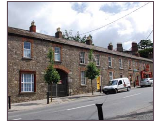
Fig.21: Early nineteenth-century terrace on north side of Church Street.
