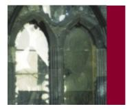
Thin polycarbonate sheeting has been used here, giving hideous "hall-of-mirrors" distortions. This can be overcome by using 6mm thick sheet, but the reflections, whilst not being distorted, will still give the building a "blind" appearance.
