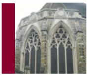
The windows at this church are fitted with stainless-steel wire-guards, but they are scarcely discernible and the visual integrity of the building has been preserved. Secondary glazing was removed prior to the fixing of the guards.
