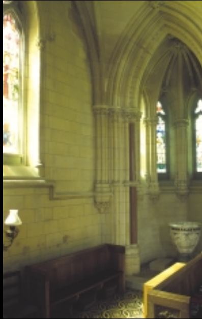
Myshall Church of Ireland Church, Co. Carlow was built by George Ashlin. It received grant-aid from the Heritage Council towards the cost of protecting the windows with stainless-steel wire-guards. The windows, by James Powell & Sons, had previously been unprotected.
