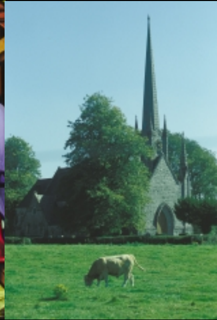
Abbeyleix Church of Ireland Church, Co. Laois was built by Thomas Wyatt and many of the windows are by Henry Holiday. It received grant-aid from the Heritage Council towards the cost of removing the secondary glazing and replacing it with stainless-steel wire-guards.
