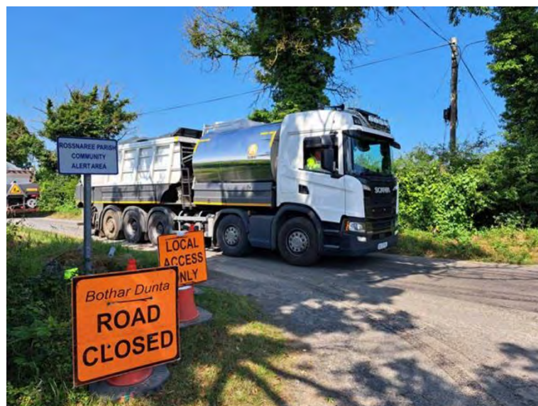
Surface dressing combination plant
