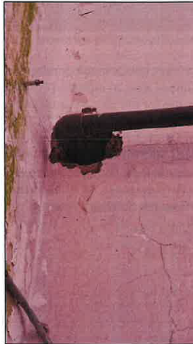
Figure 3.3 and Figure 3.4: Holes cored into walls of former handball courts. (Source: IMAC Group, 2025).
