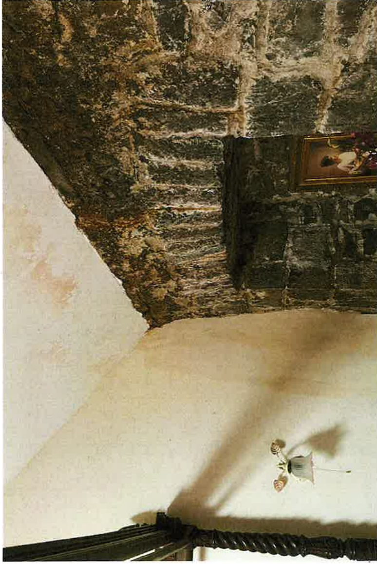
Moisture damage evident at ceiling level
