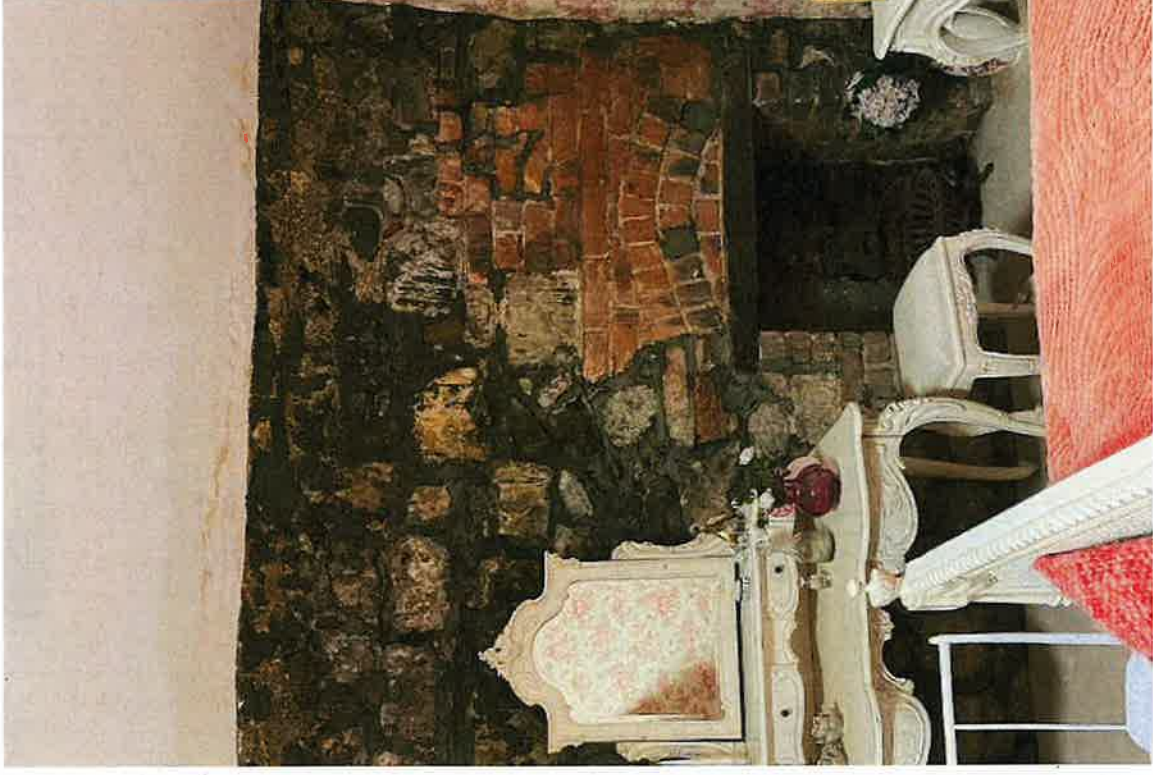
Moisture evident in mortar joints to rubble stone wall
