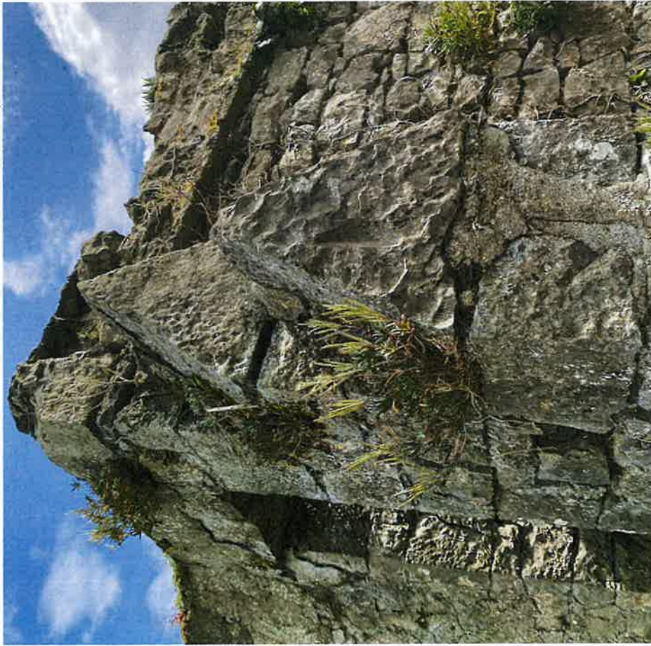
Single remaining half crenellation module showing two levels of capping, seen on western parapet
