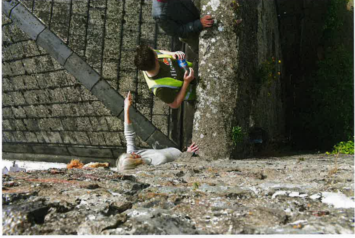
Looking down from northern turret to parapet - note cement flashing and rainwater outlet
