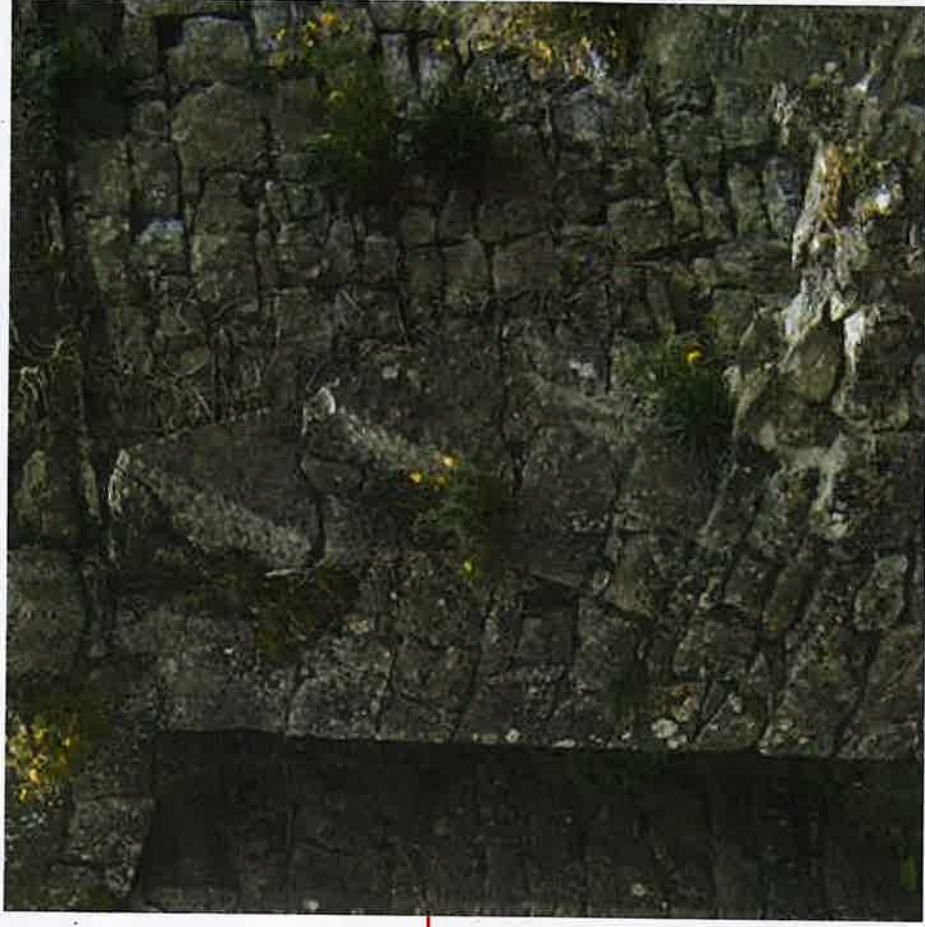
Remaining "half" crenellation to western facade with cut capping stone intact
