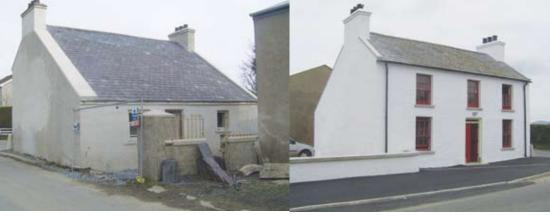
The construction of the original building is solid brickwork. This made it unusual but not unique in the district at that time. It is most likely the bricks were made on site from the fine local alluvial clay, burnt in temporary clamps. The lean-to was a very inferior construction of rubble stone.
